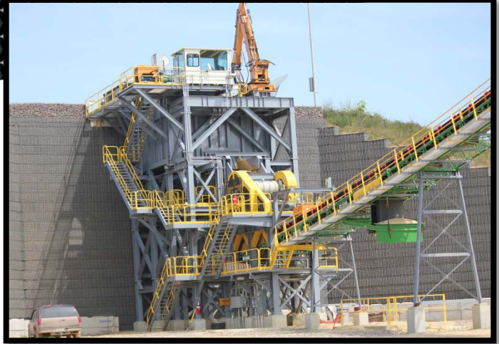
Primary Dump Hopper
