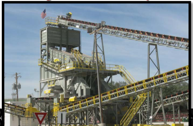
50 Ton Surge Bin & TCI Vibratory Feeders
